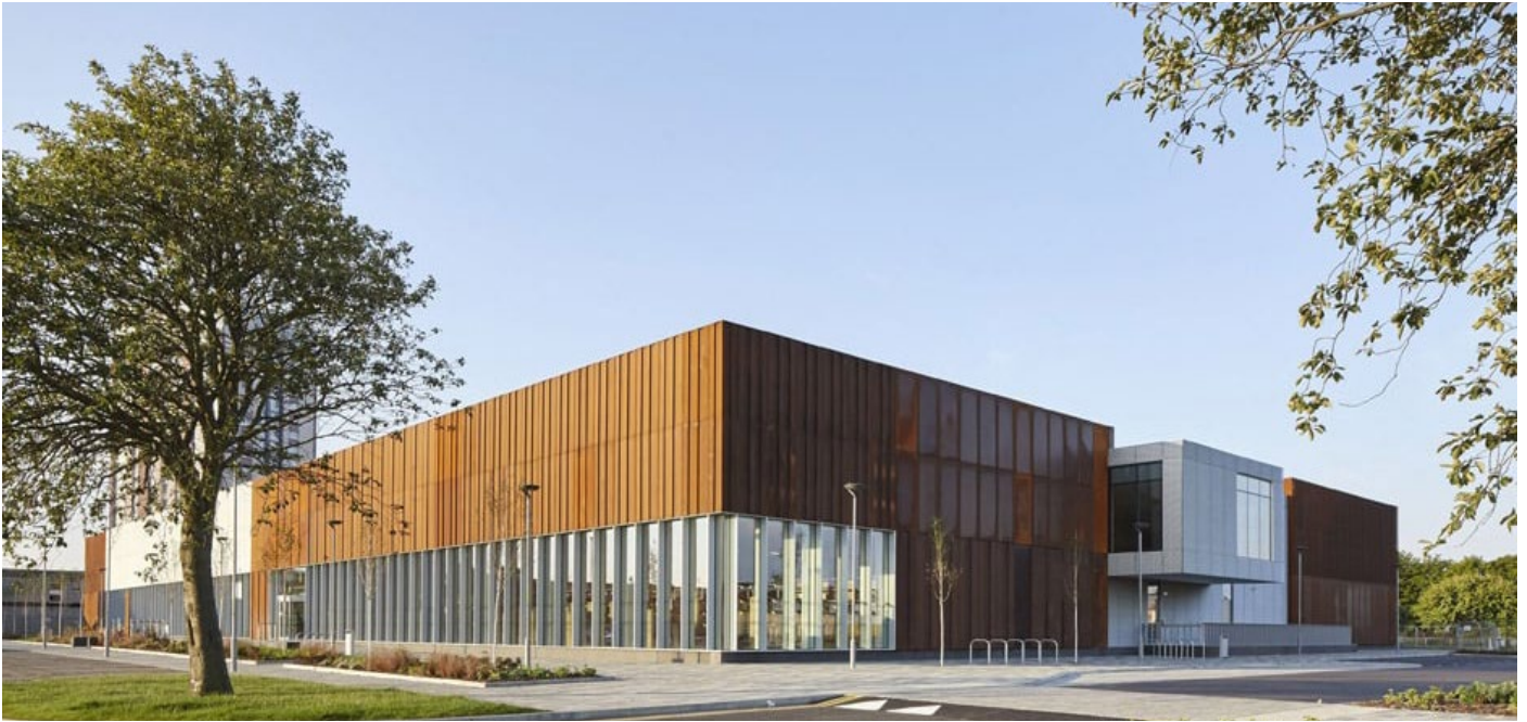
Fig. 3 Panelised core-ten façade (Faulkner Browns)
