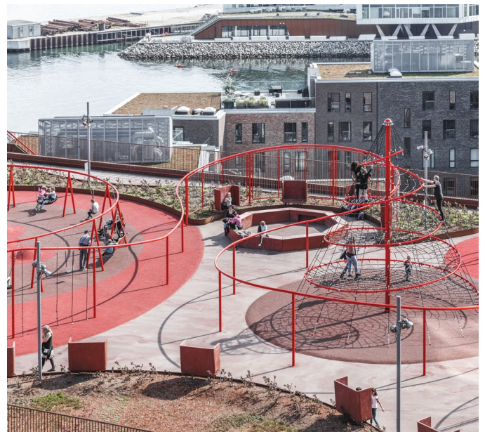
Fig. 2 Rooftop play equipment (Rasmus Hjortshøj for JaJa Architects)
